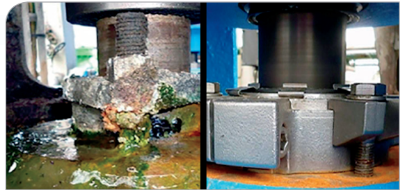
Leak-resistant mechanical seals installed to reduce maintenance needs.
