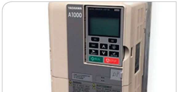
VFD drive to reduce energy costs.
